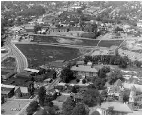
West View of Vinegar Hill After Demolition
