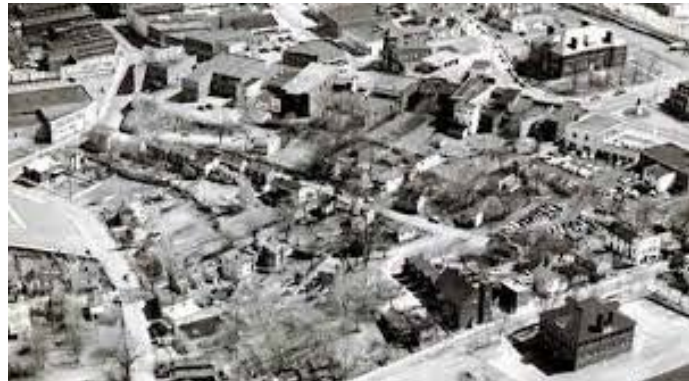
East view of Vinegar Hill before Demolition
